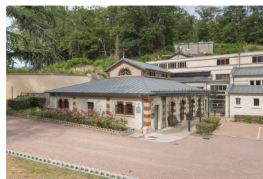
Pavillon des douches. Phot. Pierre-Marie Barbe-Richaud IVR26_20195800411NUC4A
