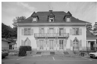
Façade sud. Phot. Jérôme Mongreville IVR43_19872501140V
