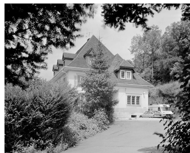
Façade est. Phot. Jérôme Mongreville IVR43_19872500288V
