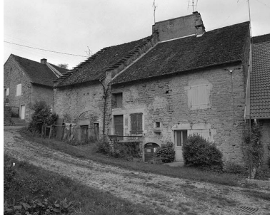
Façade droite. Phot. Yves Sancey IVR43_19813900211X
