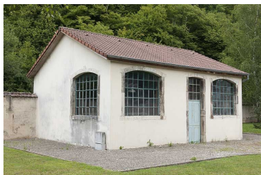
Magasin industriel. Phot. Jérôme Mongreville IVR43_20112502297NUC4A
