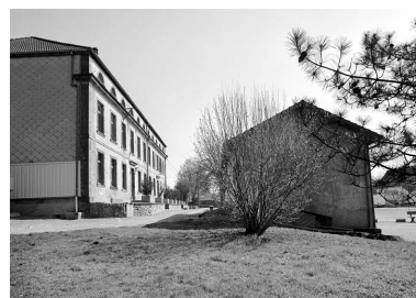
Pignons ouest. Phot. Yves Sancey IVR43_20039000078X
