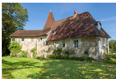
Elévation ouest. Phot. Sonia Dourlot IVR43_20167000816NUC2A
