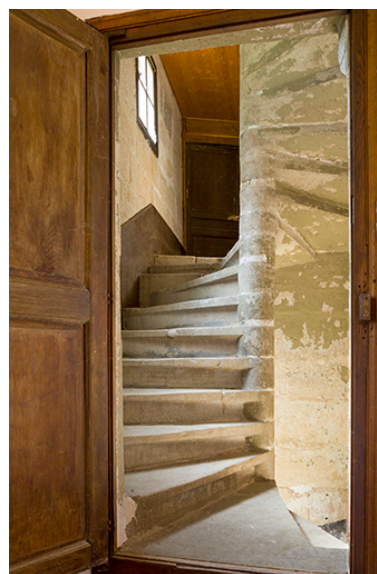
Escalier en vis. Phot. Sonia Dourlot IVR43_20167000820NUC2A
