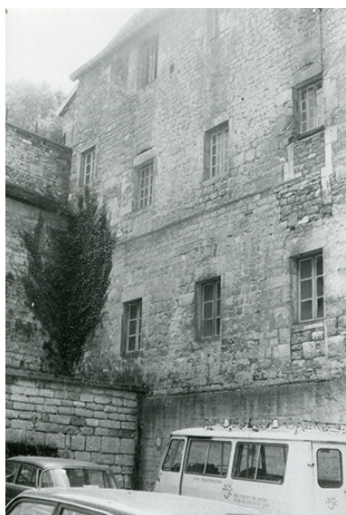
Mur nord, s.d. [vers 1970]. Phot. Georges Chenu IVR43_20243900414NUC2A
