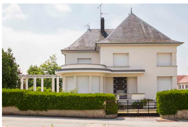
Logement patronal et pergola. Phot. Yves Sancey IVR43_20132501077NUC2A
