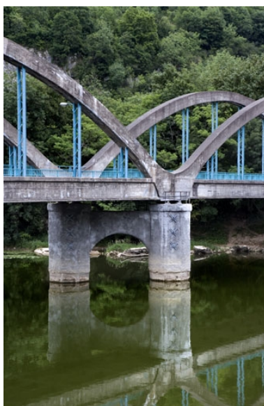
Piles centrales. Phot. Yves Sancey IVR43_20062500309NUCA
