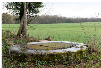
Dernier puits existant. Phot. Sonia Dourlot IVR43_20157001004NUC2A
