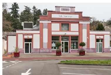
Façade. Phot. Pierre-Marie Barbe-Richaud IVR26_20227100022NUC4A
