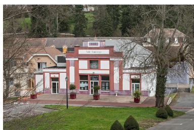
Façade. Phot. Pierre-Marie Barbe-Richaud IVR26_20227100025NUC4A
