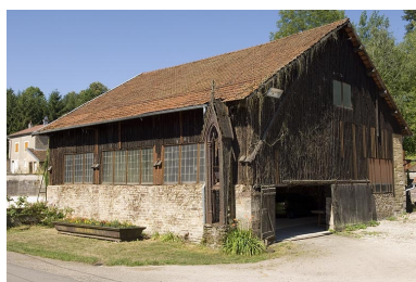
Magasin industriel. Phot. Jérôme Mongreville IVR43_20067000594NUCA
