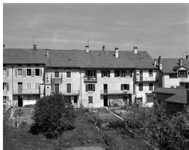
Façade postérieure. Phot. Yves Sancey IVR43_19913900331X
