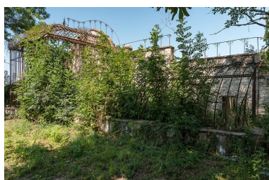
Aile est, vue de trois-quarts. Phot. Pierre-Marie Barbe-Richaud IVR26_20205800545NUC4A
