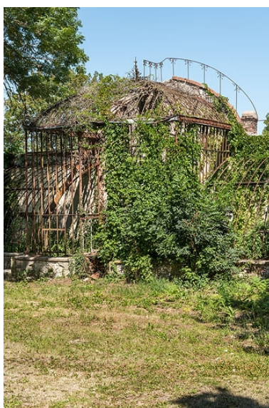
Pavillon central, vue de trois-quarts. Phot. Pierre-Marie Barbe-Richaud IVR26_20205800539NUC4A
