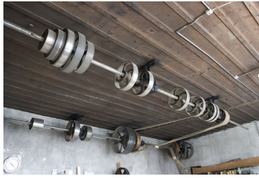
Transmissions d'un atelier. Phot. Yves Sancey IVR43_20093900111NUC2A
