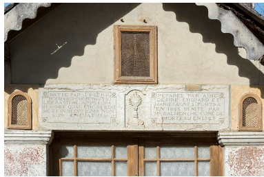
Linteau et niches. Phot. Sonia Dourlot IVR43_20172501801NUC4A
