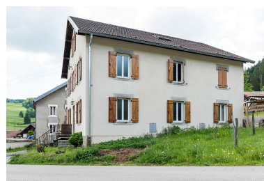
Façade latérale droite. Phot. Sonia Dourlot IVR43_20172500587NUC4A
