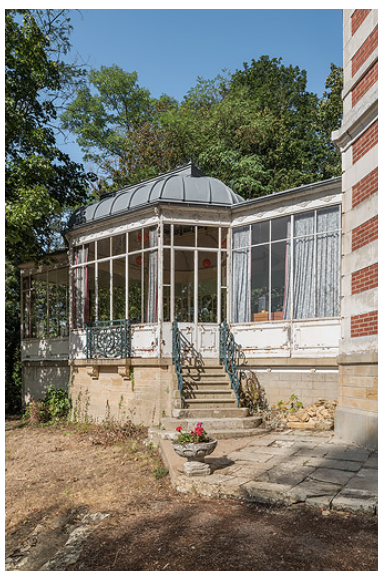
Jardin d'hiver, façade. Phot. Pierre-Marie Barbe-Richaud IVR26_20195800667NUC4A
