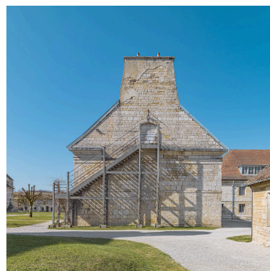
Caserne U : mur pignon est. Phot. Thierry Kuntz IVR43_20223900558NUC4A
