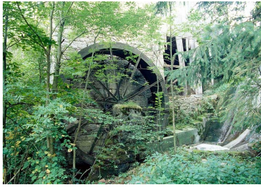
Roue hydraulique verticale. Phot. Laurent Poupard IVR43_19903900454ZA
