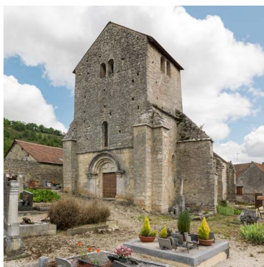
Façade principale. Phot. Pierre-Marie Barbe-Richaud IVR26_20182100116NUC2A
