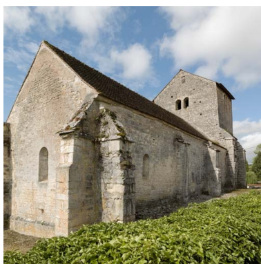
Elévation nord. Phot. Pierre-Marie Barbe-Richaud IVR26_20182100113NUC2A
