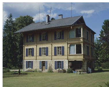
Chalet. Façade sud. Phot. Yves Sancey IVR43_20029000302XA
