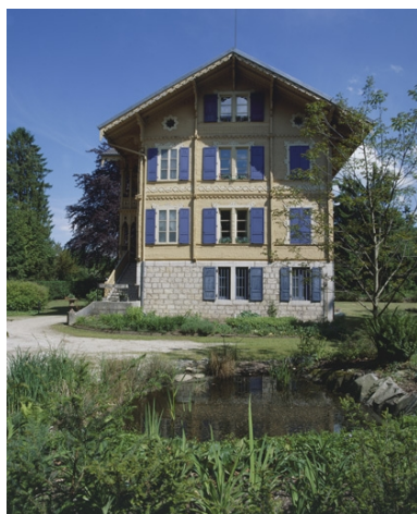
Chalet. Façade ouest. Phot. Yves Sancey IVR43_20029000304XA
