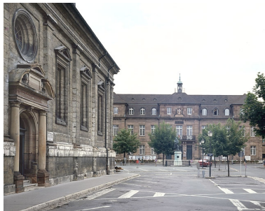
Place Saint-Martin. Phot. Jérôme Mongreville IVR43_19882500175VA
