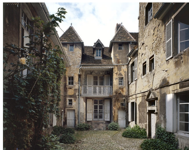
Façade antérieure. Phot. Yves Sancey IVR43_19883900105VA
