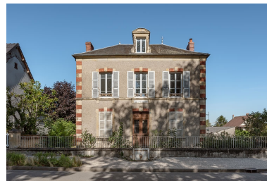
Façade principale. Phot. Pierre-Marie Barbe-Richaud IVR26_20205800506NUC4A
