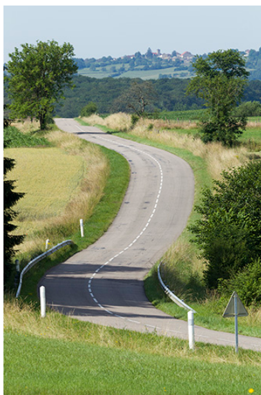
La route départementale 434. Phot. Sonia Dourlot IVR43_20157001051NUC2A
