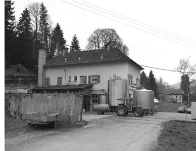
Façade nord. Phot. Yves Sancey IVR43_19973900638X
