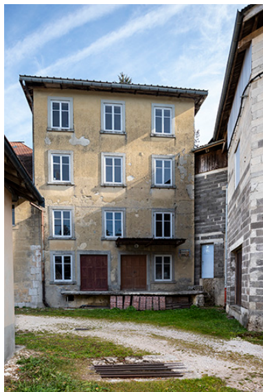
Minoterie. Phot. Sonia Dourlot IVR43_20182501712NUC4A
