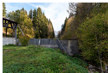
Bassin de retenue. Phot. Sonia Dourlot IVR43_20182501717NUC4A
