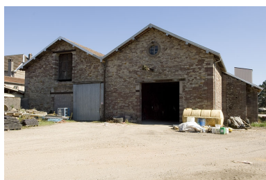
Murs-pignons nord. Phot. Jérôme Mongreville IVR43_20067000588NUCA
