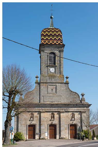
Façade principale. Phot. Jérôme Mongreville IVR43_20177000215NUC4A
