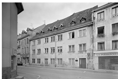
Façade principale. Phot. Jérôme Mongreville IVR43_19872501125V
