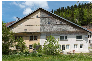
Façade postérieure. Phot. Sonia Dourlot IVR43_20172500648NUC4A
