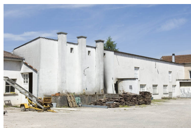
Salle de distillation moderne. Phot. Jérôme Mongreville IVR43_20097000325NUC2A
