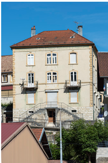
Façade antérieure. Phot. Sonia Dourlot IVR43_20162500916NUC4A
