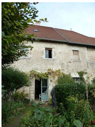
Façade sud Phot. Sabrina Dalibard IVR43_20137000862NUC2A
