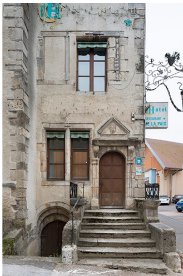
Façade principale. Phot. Jérôme Mongreville IVR43_20177000685NUC4A
