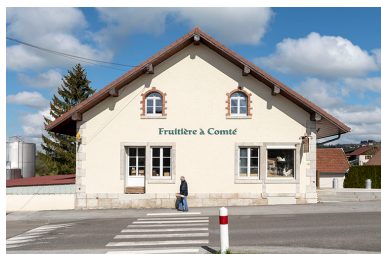
Façade antérieure. Phot. Sonia Dourlot IVR43_20192500617NUC4A
