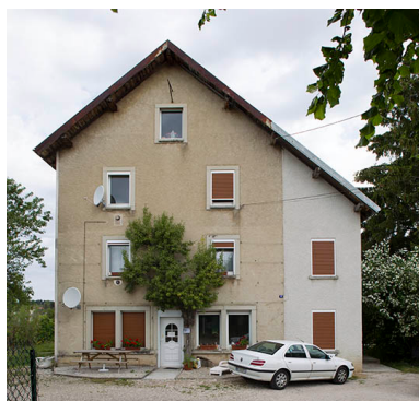
Façade antérieure. Phot. Sonia Dourlot IVR43_20142501866NUC4AQ
