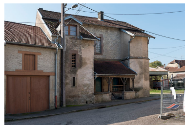
Façade antérieure. Phot. Sonia Dourlot IVR43_20157001400NUC4A
