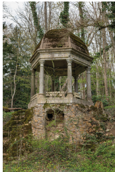
Face ouest. Phot. Pierre-Marie Barbe-Richaud IVR26_20245800152NUC4A
