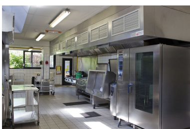
Restauration : la cuisine. Phot. Yves Sancey IVR43_20122500762NUC2A
